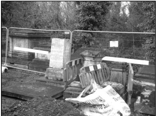
Monument repairs in progress January 2019. Photo: Jeff Hart
