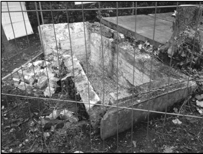
The Lewis grave filled with pea gravel before reconstruction work begins
