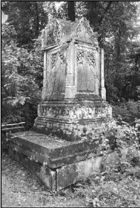
Wallbuton monument before restoration.
