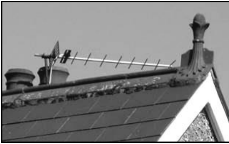
Modern replacement on modern roof
