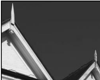
Well maintained finial
