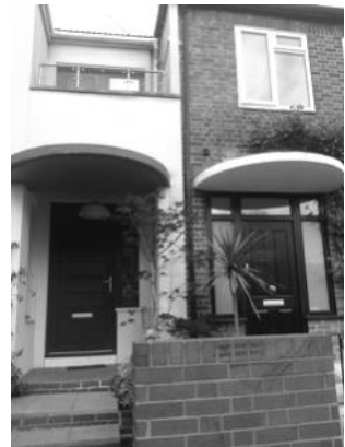
Fig 8. 'Modernist' in-fill houses on the Dollis Hill Estate with porches - one recessed door and one in-filled porch
