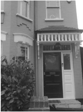
Fig 7. A 'simple' un-recessed porch on the Dollis Hill estate
