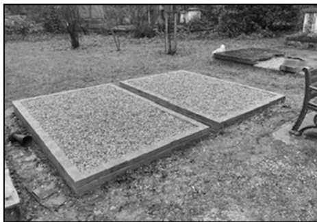
Before and after: Two damaged vaults with gaping holes on the west side of the chapel now marked with low brick kerbing and filled with gravel. Photos: Jeff Hart
