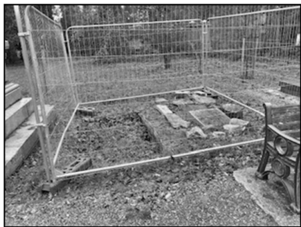
Before and after: Two damaged vaults with gaping holes on the west side of the chapel now marked with low brick kerbing and filled with gravel. Photos: Jeff Hart
