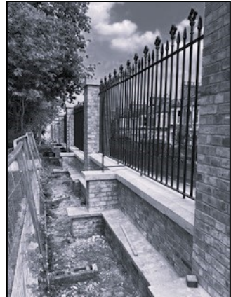
(1) East wall showing final curved railing gap to be completed prior to safety barrier removal.
