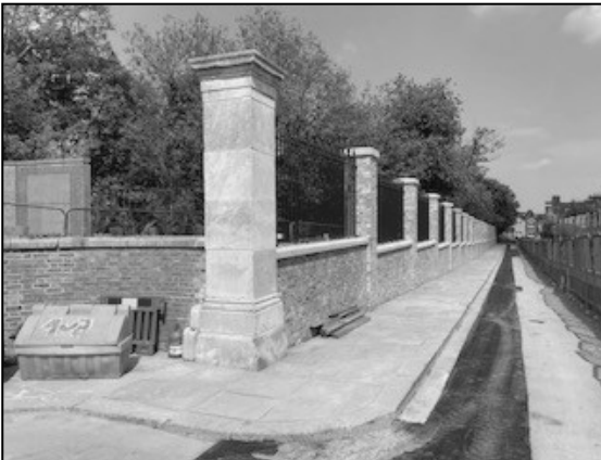
(1) East wall showing final curved railing gap to be completed prior to safety barrier removal.
